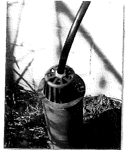
7. Drain is installed outside the home to prevent flooding in the event system ever fails.
