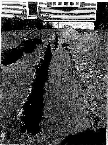
2. Trench area for system.
